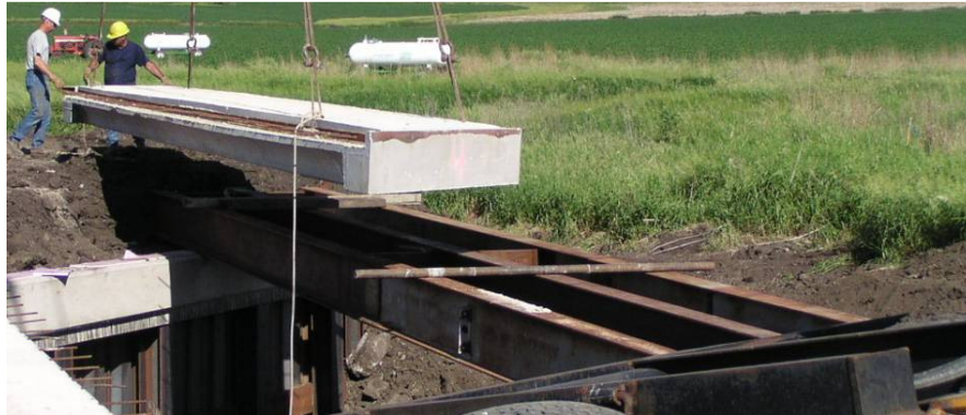
Figure 70. Temporary beams for setting panels.
