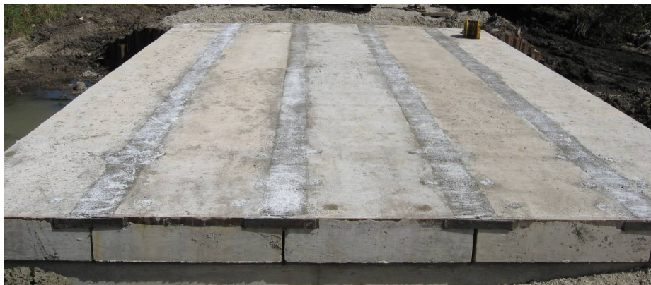
Figure 81. Concrete in closure area.
