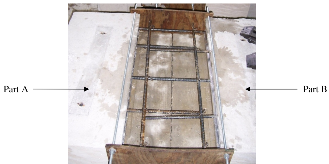
Figure 20. Position of reinforcing bar before closure.
