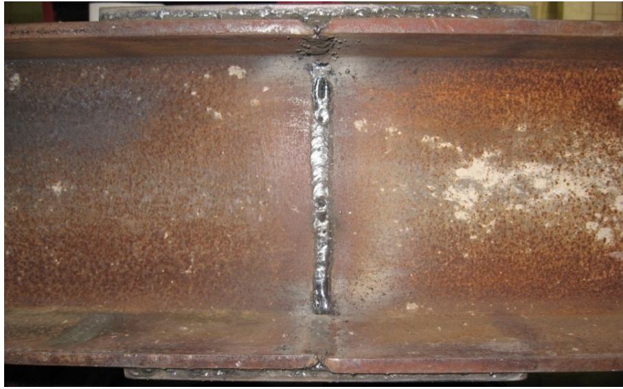
Figure 64. Repaired H-pile splice.
