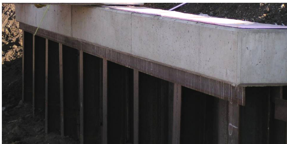
Figure 69. Abutment cap on H-piles.
