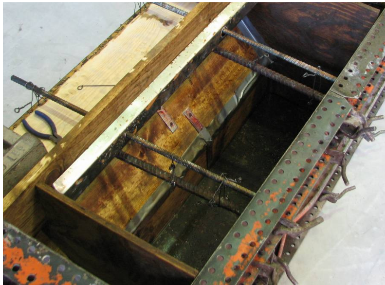
Figure 18. Photograph of reinforcement in forms.
