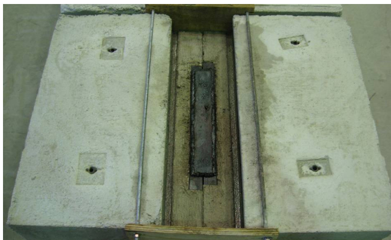
Figure 25. Type 2 Connection prepared for closure pour.
