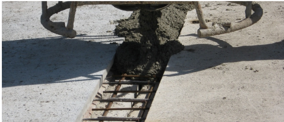
Figure 80. Using concrete bucket for placement.
