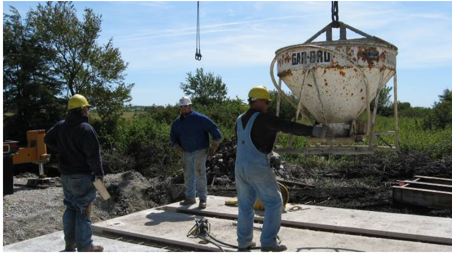
Figure 80. Using concrete bucket for placement.
