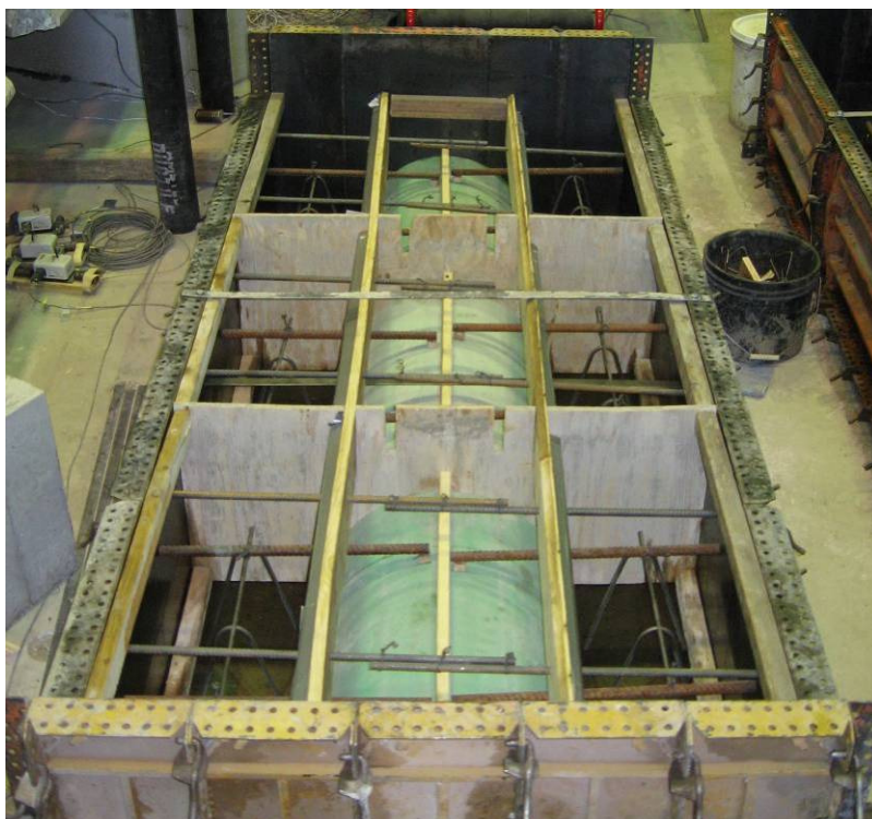
Figure 27. Completed formwork for Type 3 Connection.
