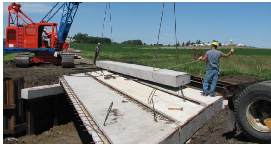
Figure 72. Setting panel on superstructure.
