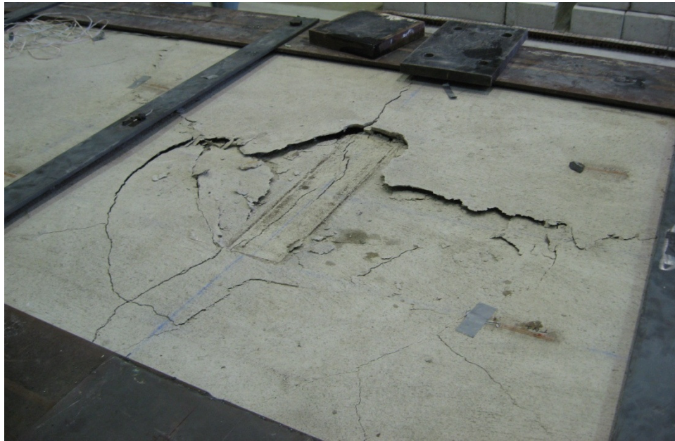
Figure 66. Failed abutment backwall specimen.
